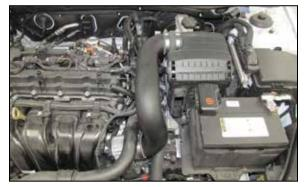
15. Install the intake tube assembly into the coupling hose at the throttle body and then into the hose at the air box, secure the tube with the provided hose clamps.
