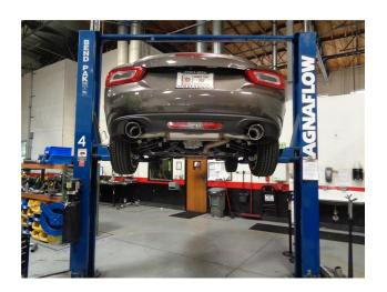
**Step 4.** Once a final position has been chosen for the new exhaust system, evenly tighten all clamps from front to rear using the torque specifications on page one of the instructions. Re-install the underbody X-Brace. Inspect all fasteners after 25-50 miles of operation and re-tighten if necessary.
